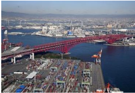
(a) Minato Cantilever Truss Bridge
