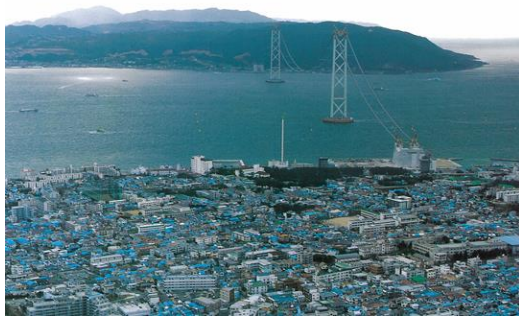
(a) Akashi-Kaikyo Bridge after 1995 Kobe Earthquake
