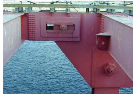
(b) Movement at the pin connection
