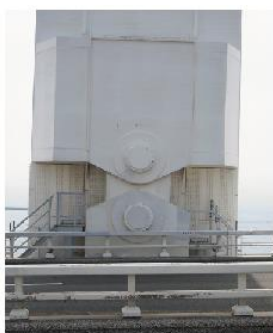
Fig. 8 Photo of LBC at tower of Yokohama-Bay Bridge and Monitoring system and observed seismic record at 2011 Tohoku Earthquake. (a) accelerations of tower at deck level during the main shock showing spike indicating impulses (b) time interval between successive lateral poundings (Siringoringo et al. 2013)
