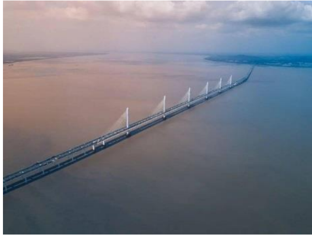
Fig. 4 Photograph of the Jiashao Bridge
