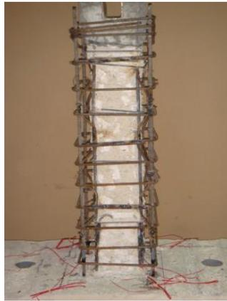
(b) welding of lap splices in the original column and R/C jacket reinforcement
