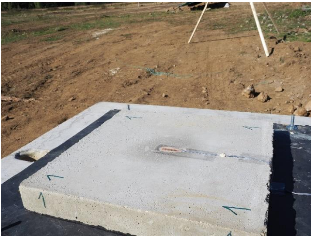
Fig. 5 Strain gauge placed on the top surface of the concrete slab
