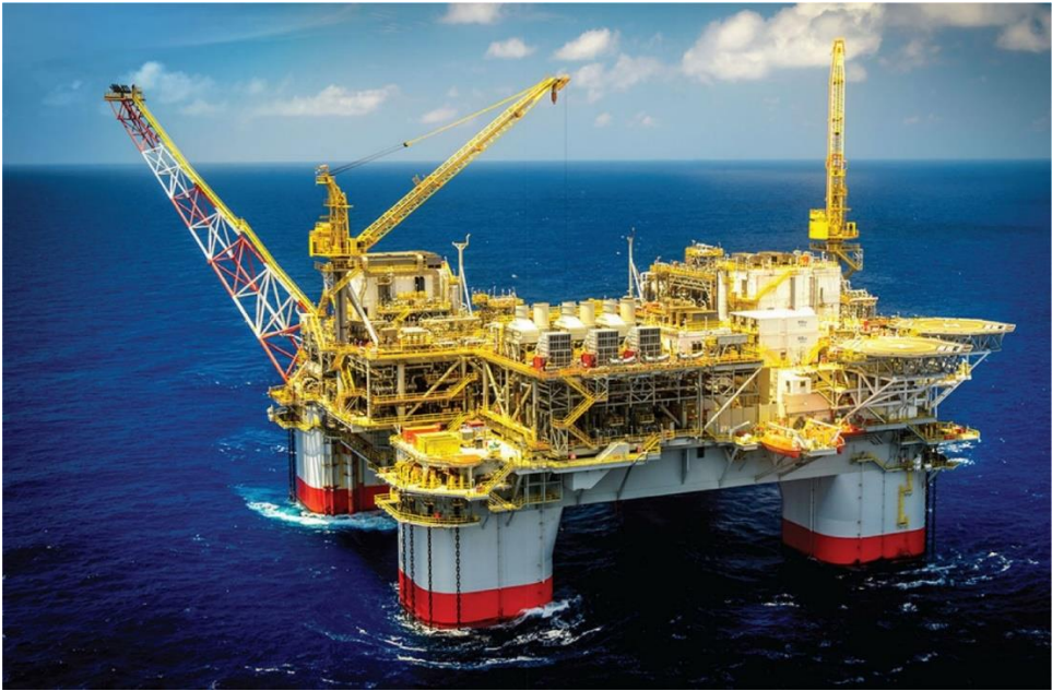
Fig. 13 Completed Jack and Saint Malo (JSM) in actual operation
