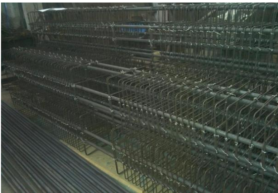
(a) Reinforcement skeleton of column
