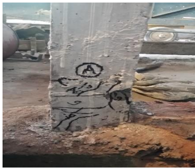
(e) Cracks in Column Hinge A
