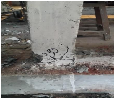
(g) Cracks in Column Hinge C
