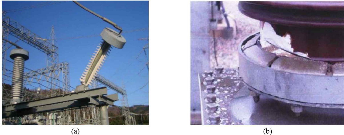
Fig. 1. a) Damaged lightning arrester after Fukushima earthquake (2011) (Tokyo Electric Power 2011); b) Leakage in capacitive transformer during Bam earthquake (2003) (Karami-Mohammadi et al. 2019)
