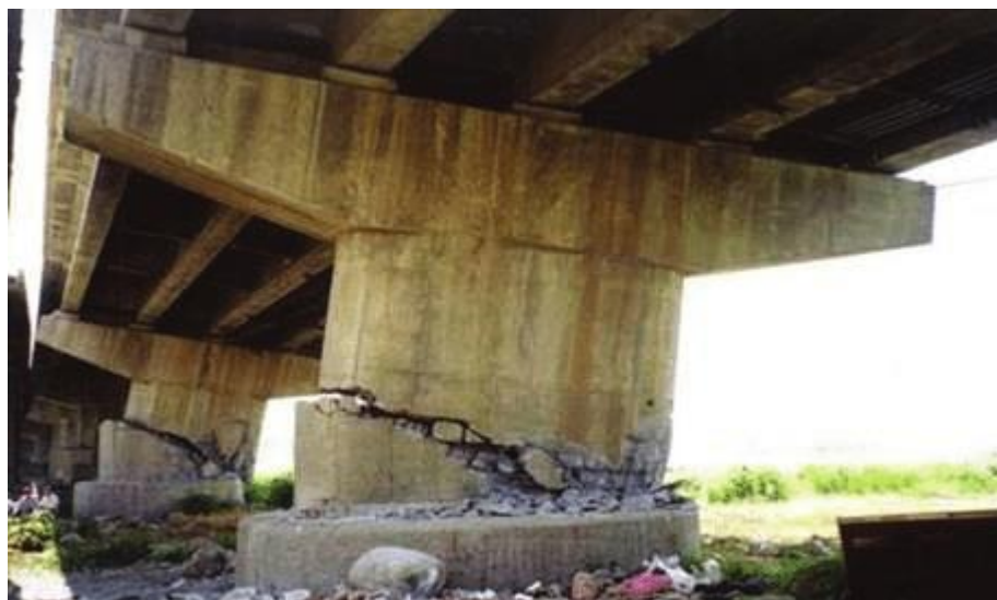
Fig. 3 Some permanent damages on the Wu-Shi Bridge wall pier after the Chichi earthquake (Sung et al. 2009)
