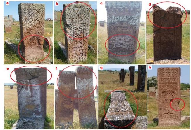
Fig. 4 The damage observed in gravestones: a) loss of mass, b) lichen formation, c) calcification, d) breaking damage, e) cracking damage, f) vertical displacement, g) tipping damage, h) partial loss
