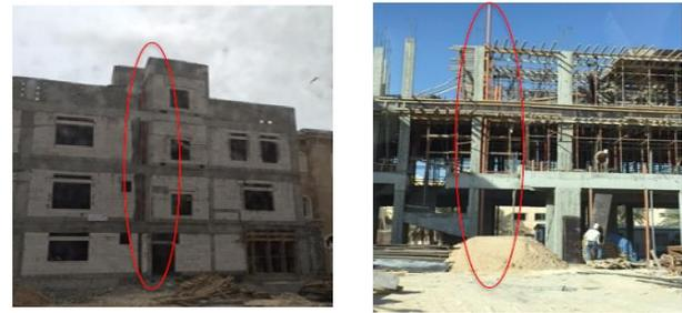
Fig. 3 Service pipes installed through vertical openings in the RC beams in a typical residential building in Kuwait
