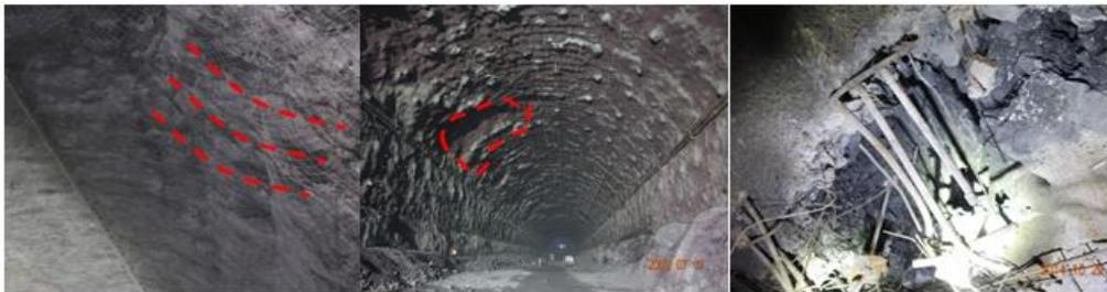
(a) Upstream arch shoulder rock drum (b) Poor upstream molding (c) The rib arch of upstream side arch is bent
