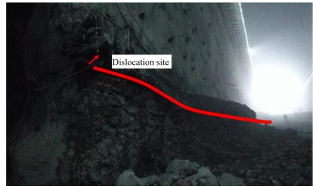
Fig. 15 Macroscopic deformation form after completion of  $C_2$  excavation
