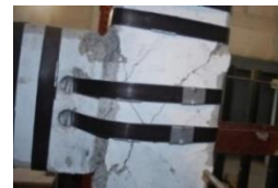
(c) cracking at joint core
