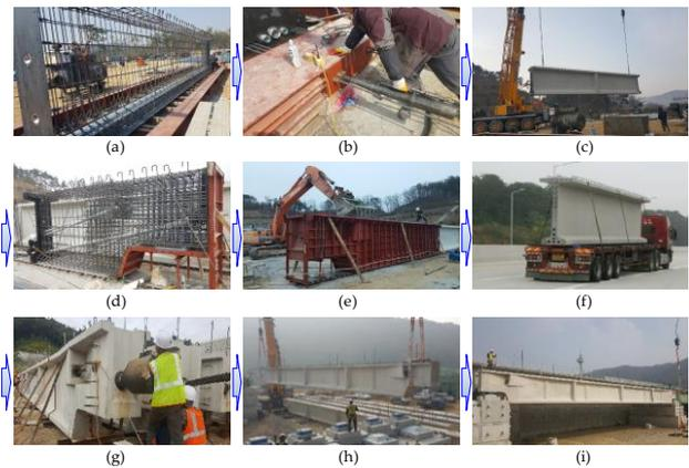
Fig. 16 Fabrication and application procedure of HPSC girder; (a) installation of rebars for mid-segment, (b) pre-tensioning of PS strands before concrete placing, (c) completion of mid-segment through concrete placing and detensioning, (d) installation of rebars and sheath for outside-segment, (e) concrete placing and curing of outside-segment, (f) carrying segments to field, (g) combining segments by post-tensioning, (h) erecting HPSC girder, (i) completion of application
