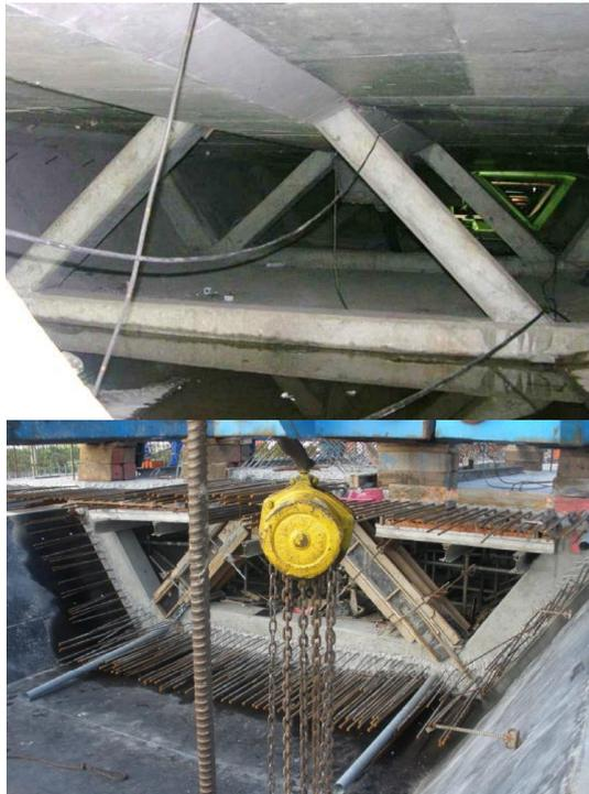
Fig. 16 Internal view of a strengthening W-section (GOMES 2013 and TOLEDO 2014)
