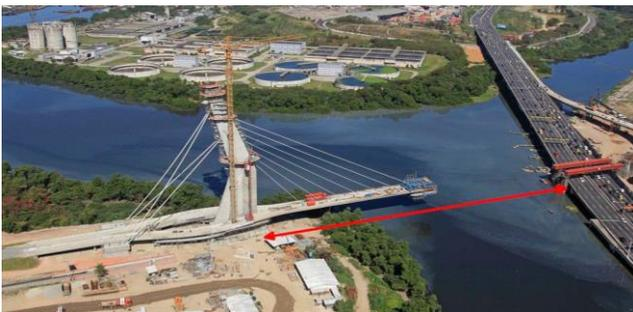
Fig. 17 Cast in place segmental cantilever method (GARAMBONE 2012)
