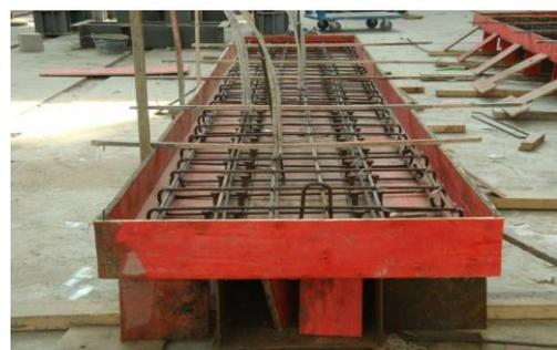
Fig. 2 Fabrication procedure of composite girders
