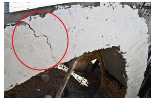
(a) Cracks in an intermediate point on the opposite side of the load
