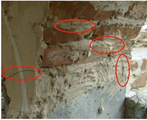
(a) Cracks at the closest point to the spring
