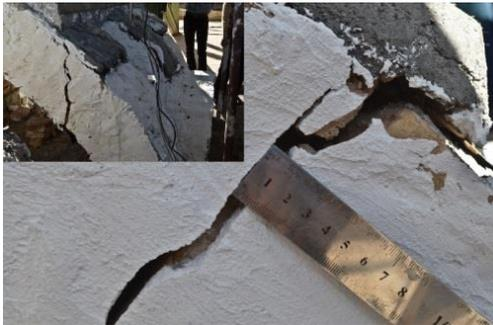
(b) The width of the cracks in the vault
