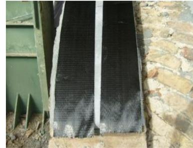
(b) Installing CFRP
