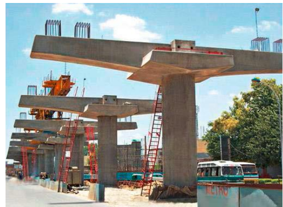
Fig. 1 Pier cap of Delhi metro train project
