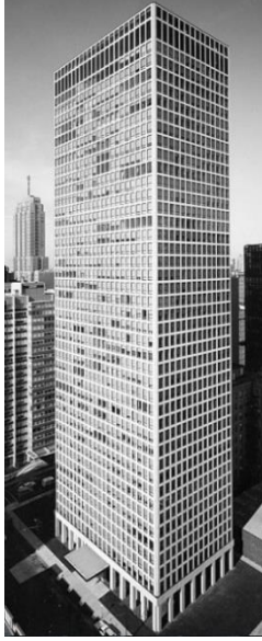
Fig. 1 Framed-tube system used in Dewitt Chestnut building
