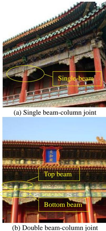
Fig. 1 The joints of ancient architecture
