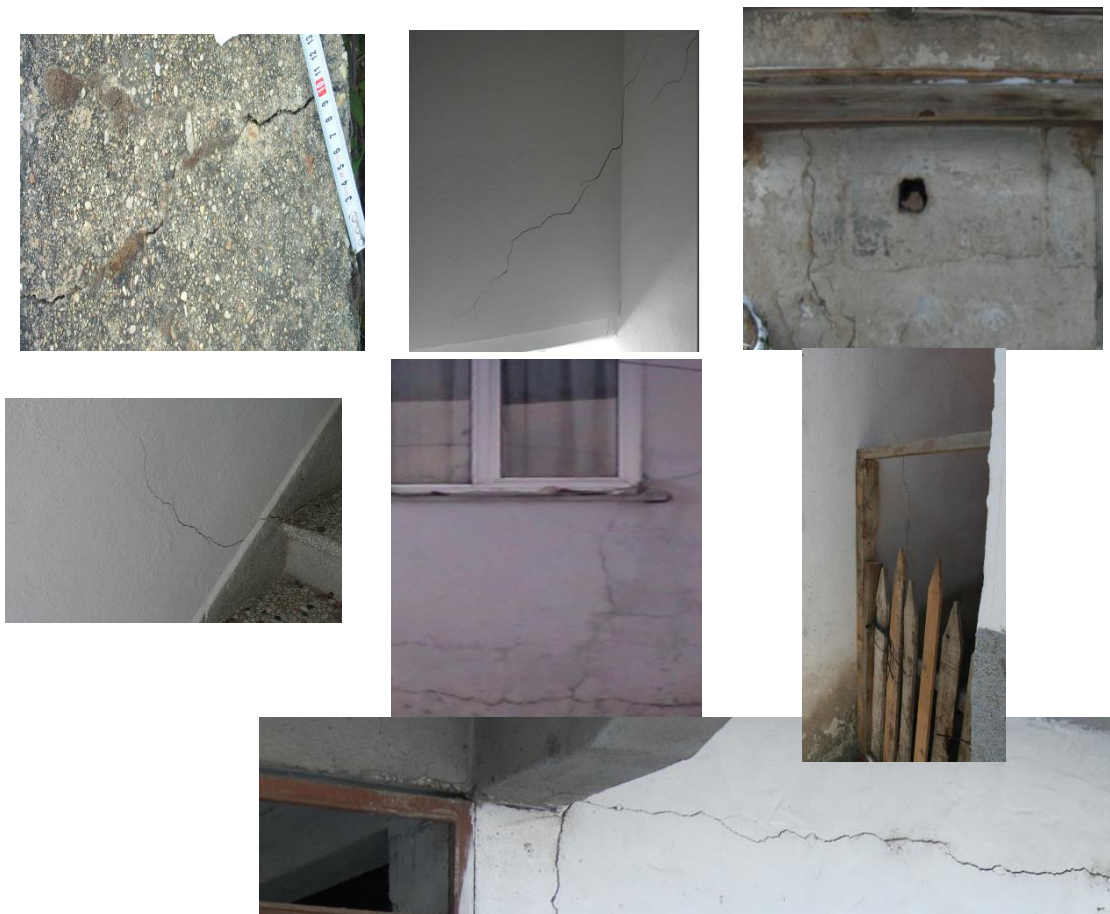
Fig. 9 Damages in some village house, located 500 m away from the mine
