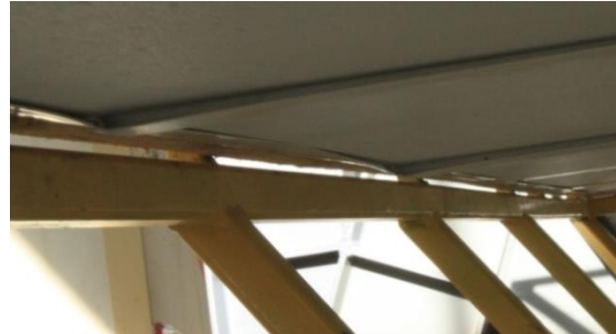
(b) Low-level crushing of a moulding (from config. 2, see Table 2)
