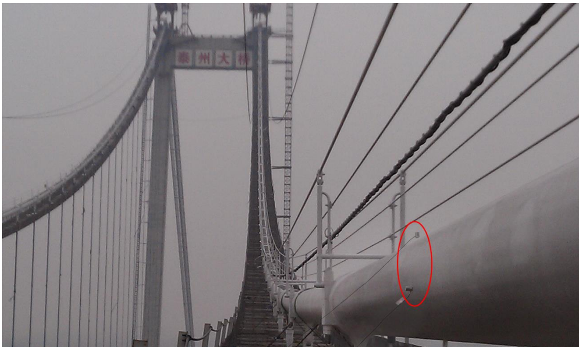
Fig. 7 Accelerometers mounted on the main cable
