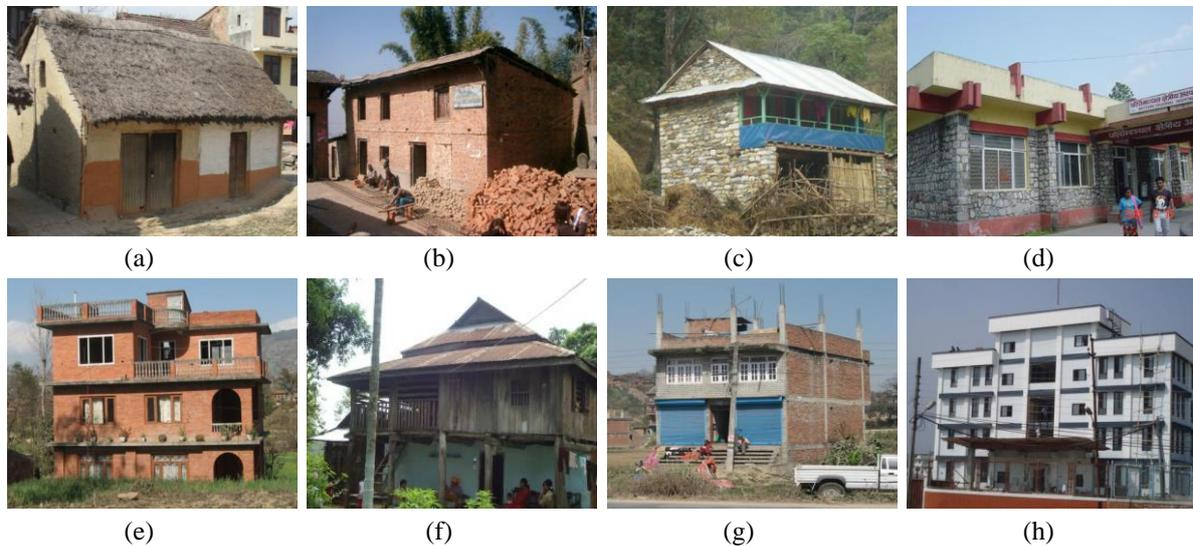
Fig. 3 Existing building typologies in Nepal: (a) Adobe, (b) Brick in mud mortar, (c) stone in mud mortar, (d) Brick in cement mortar, (e) Stone in cement mortar, (f) Wooden, (g) Non-engineered building, and (h) Engineered building
