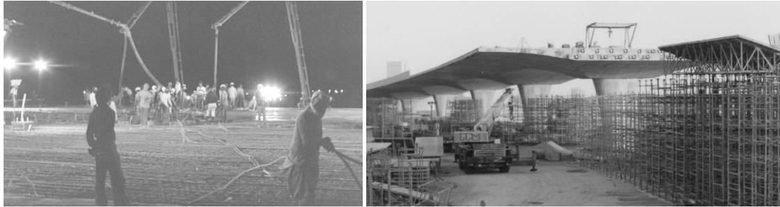
Fig. 17 Bridge construction. (a) Casting by night, (b) Completed spans and continuous scaffolding for the formworks
