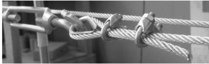
Fig. 4 Anchoring detail of the wire rope connection: stretcher, thimble and clips
