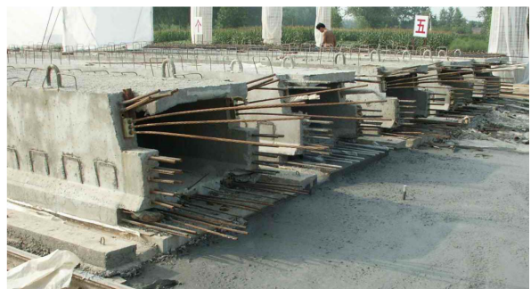
Fig. 2 Post-tensioned voided slab girders with flat anchorage
