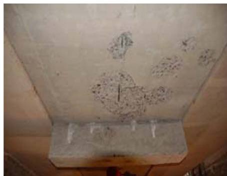
Fig. 5 Spalling on the bottom of slab
