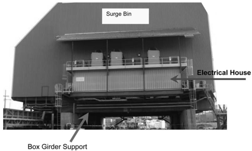
Fig. 1 Surge bin facility supported by box girders
