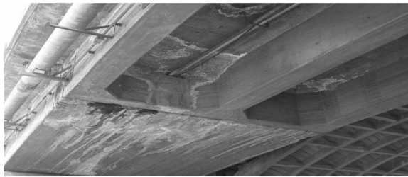
Fig. 11 Corrosion of main beam
