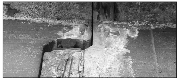
Fig. 12 Corrosion of bearing steel plates and shift
