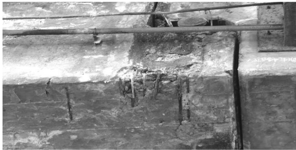
Fig. 13 Damages of corbel
