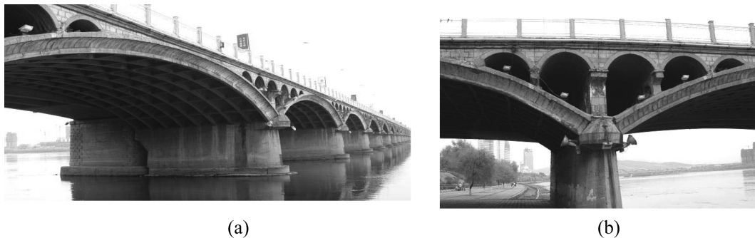
Fig. 1 Jilin highway concrete bridge (a) longitudinal view of bridge holes, (b) spandrel arch and pier view
