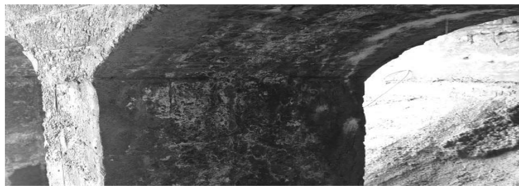
Fig. 7 Cracks damages of pier and pier caps of spandrel arch
