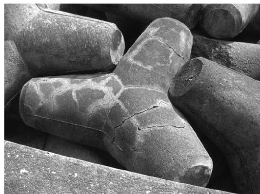
Fig. 10 Cracked tetrapod
