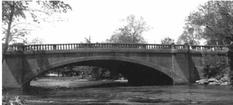
Fig. 1 A typical single span bridge having symmetrical parabolic haunches
