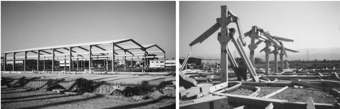
Fig. 2 The state of the building before and after the Kocaeli Earthquake-1999 (Arslan 2006)
