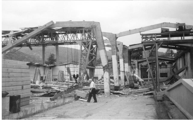
Fig. 3 Overall collapse of the prefabricated systems
