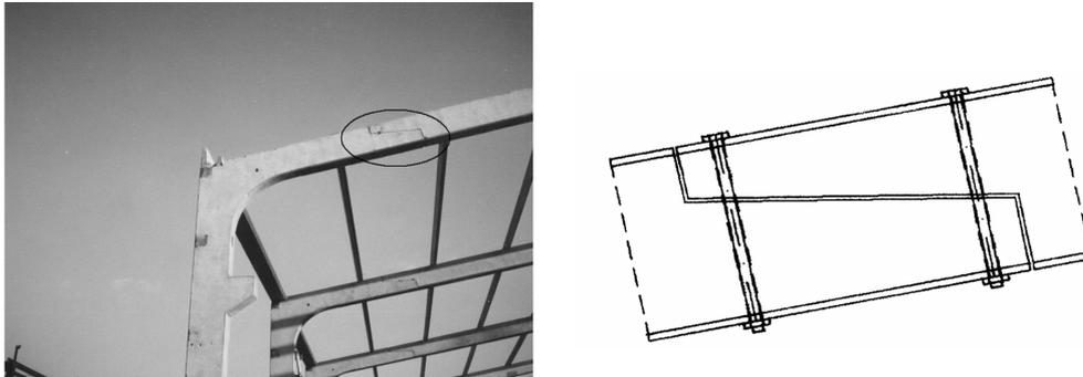
Fig. 8 Scarfed joint of a prefabricated industrial plant
