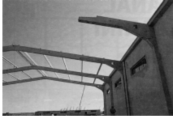
Fig. 1 View of structure being enlarged by a bolted beam connection
