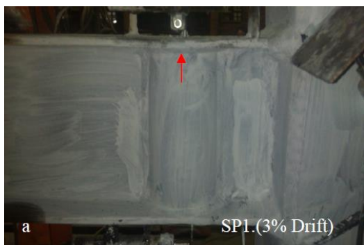
(a) Local buckling in the right beam at 3% story drift
