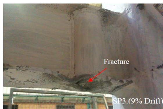
(f) Fracture in the right beam at 9% story drift
