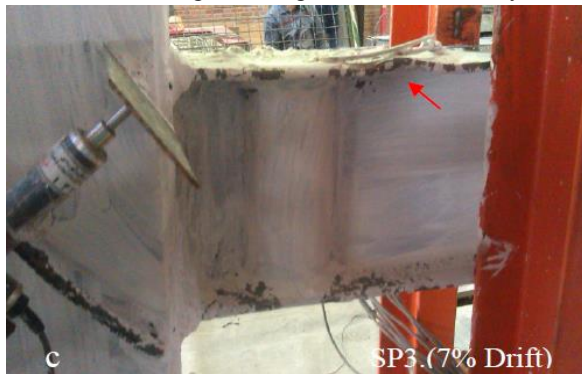
(c) Lateral-torsional buckling in the left beam at 7% story drift
