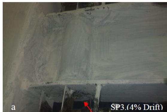
(a) Local buckling in the right beam at 4% story drift
