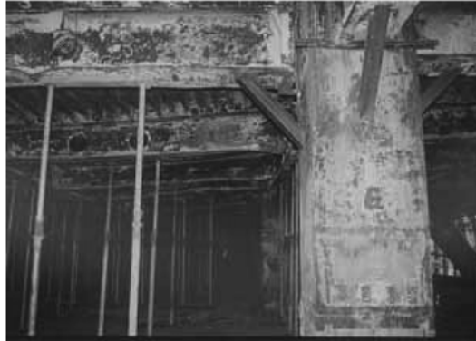
Fig. 1 Damage to beam-column connection of a tower steel building in Taipei Science and Technology Park
