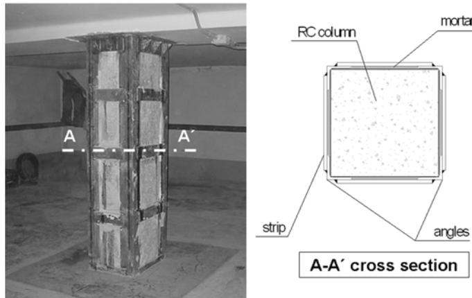
Fig. 1 Example of RC column strengthened by steel angles and strips
