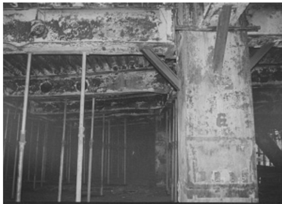
Fig. 2 Damages to the connections in TaiPei Science and Technology Park
