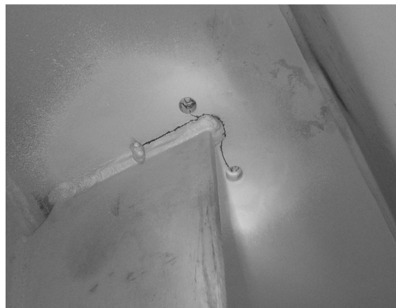
Fig. 2 Fatigue crack at the top of a vertical stiffener in steel bridge
