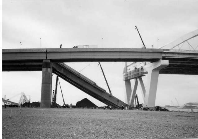
Fig. 1 Collapse of a steel bridge due to earthquake
