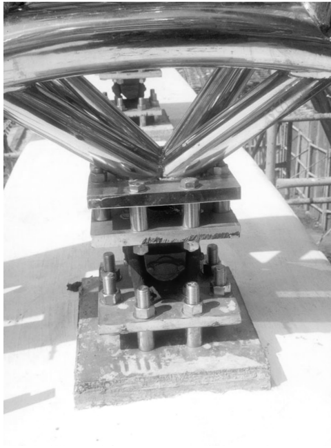
Fig. 15 Bearing detail
