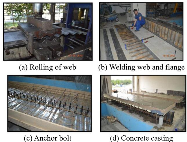
Fig. 4 Fabrication processes of composite corrugated web beams
