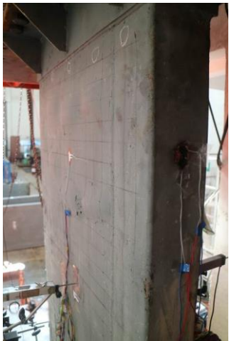
(b) Failure on side N Continued-
