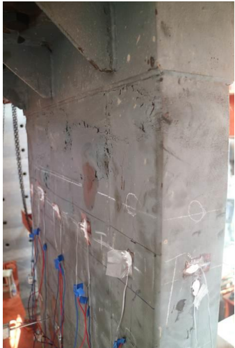
(a) Failure on side S
