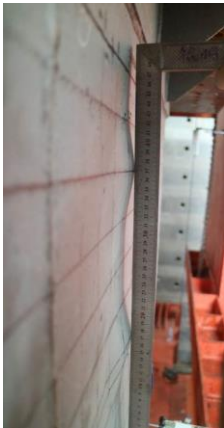
(a) Buckling of upper half of wall height
