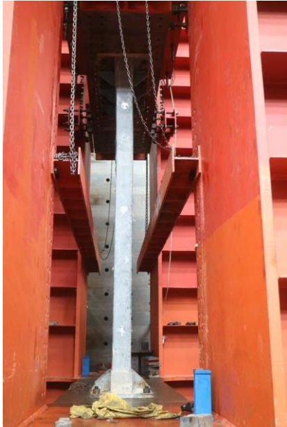
(b) Failure on side E
