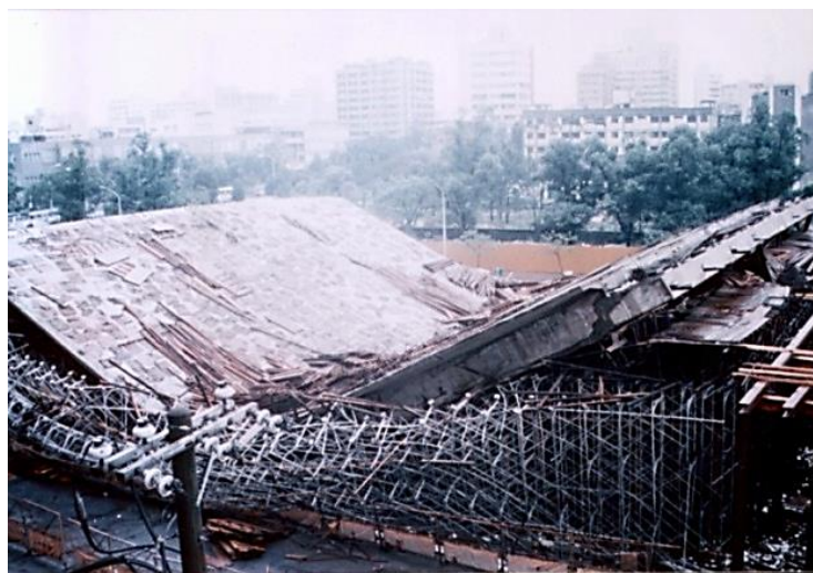
Fig. 2 Collapse of a combined system of scaffolds and shores in Taipei, Taiwan (provided by Professor Jenn-Chuan Chern at National Taiwan University)
