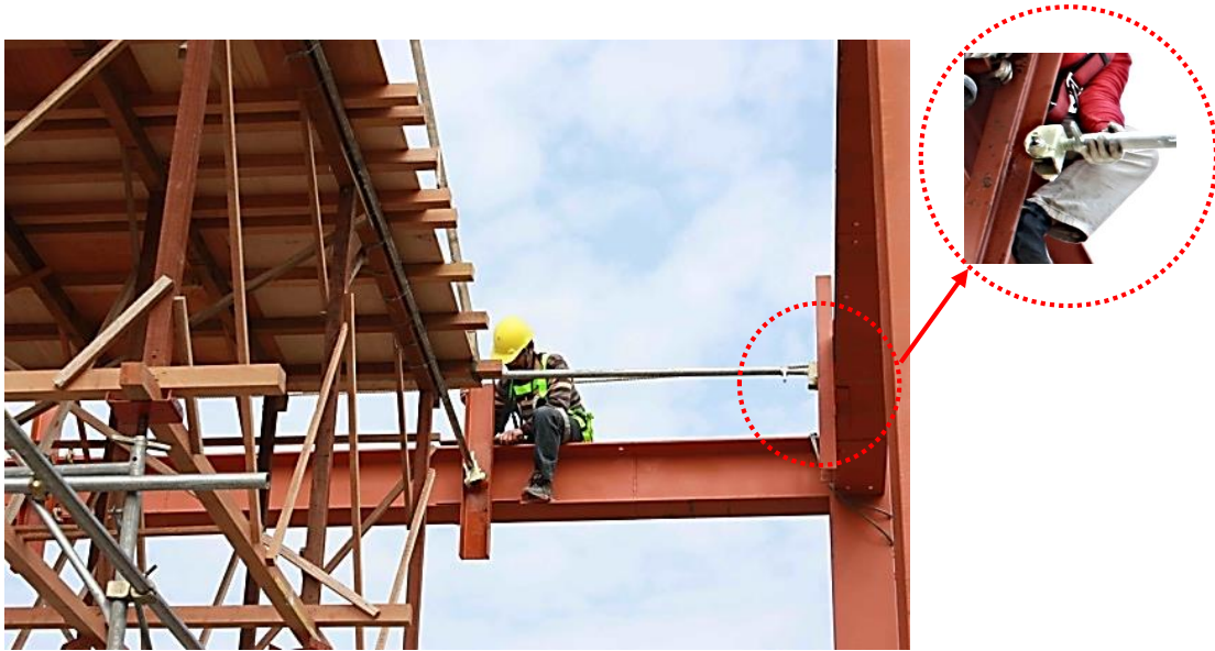
Fig. 6 Lateral bracing at the top formwork in the outdoor loading test of the combined system of scaffolds and shores
