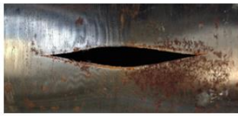
(a) Intact pipe
