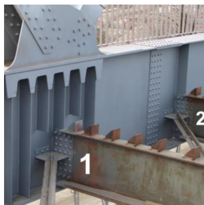
Fig. 1 Location of cross-beams in a modern through truss bridge
