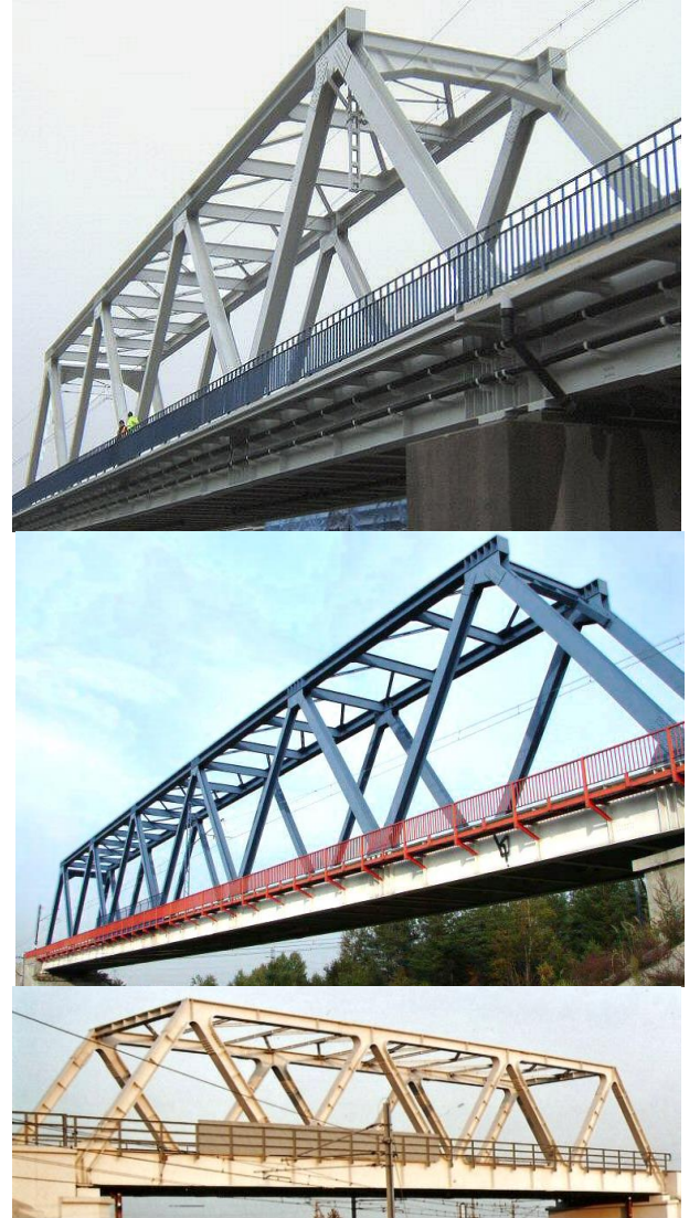
Fig. 10 The analyzed through truss bridge spans: Span-51 (top), Span-93 (middle), Span-38 (bottom)
