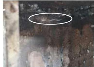
(f) Partial fracture at link web to beam connection
