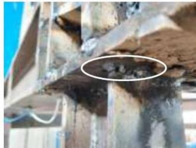
(e) Welding seam breakage at link flange to beam connection
