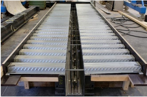
(a) Steel decks in the formwork nailed on the U-shaped beam
