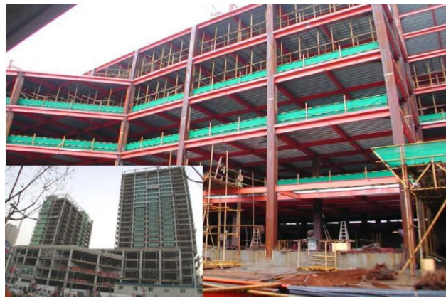
Fig. 2 Lateral resisting frame system with CFT column (Han et al. 2014)
