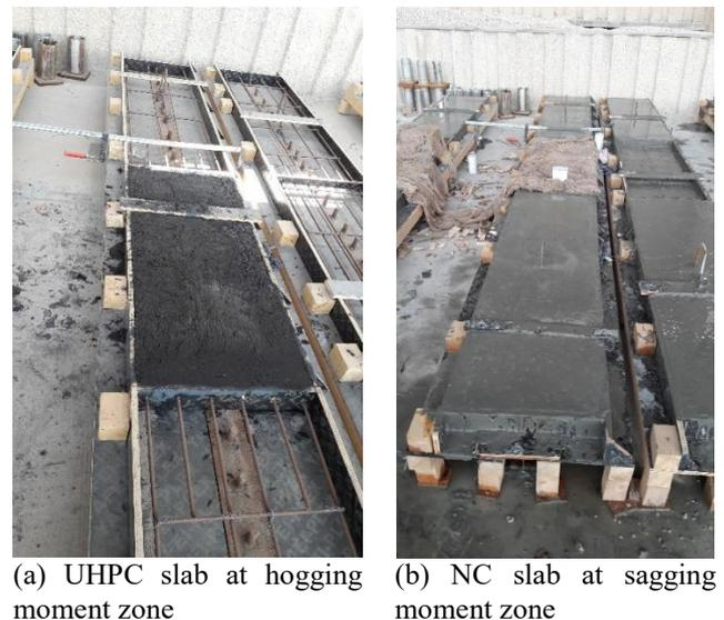
Fig. 2 Casting of concrete slabs
