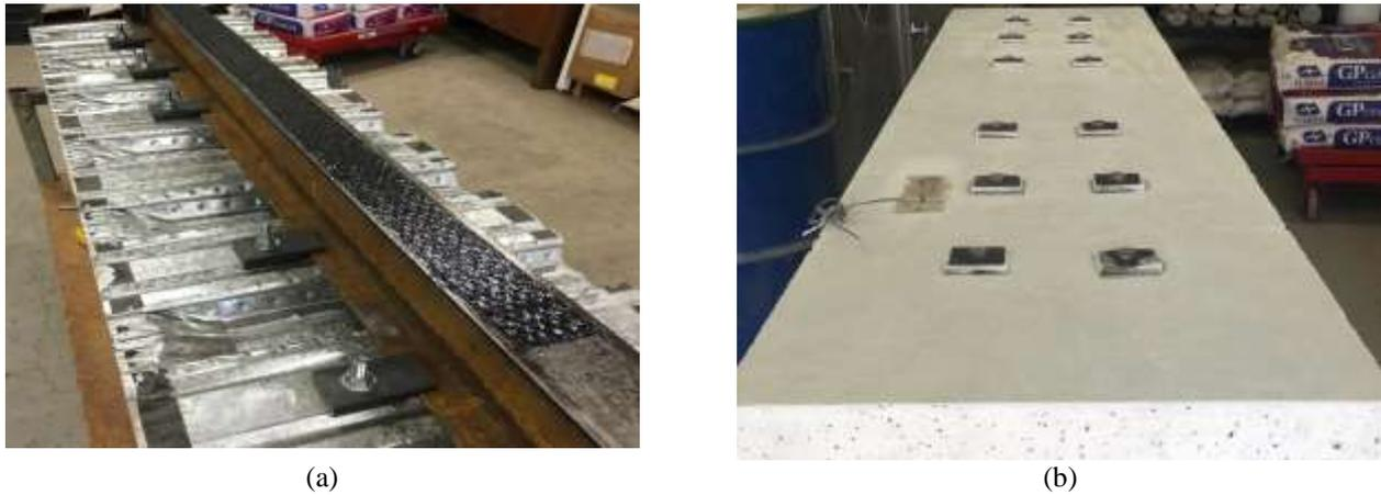
Fig. 7 (a) Strengthening of Beam 6 (upside down) and (b) top view of longitudinal shear strengthening
