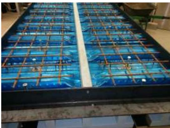
Fig. 3 Rebar arrangement of composite beams (2 beams were cast together)
